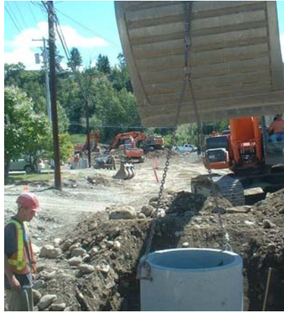
Sewer work in Kelowna, 2005.
